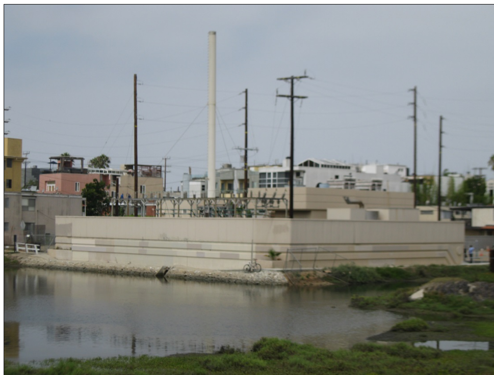
Looking northwest at 140 Hurricane Street: Venice Pumping Plant. View from Via Dolce. Photo taken on August 19, 2015 (ICF).
