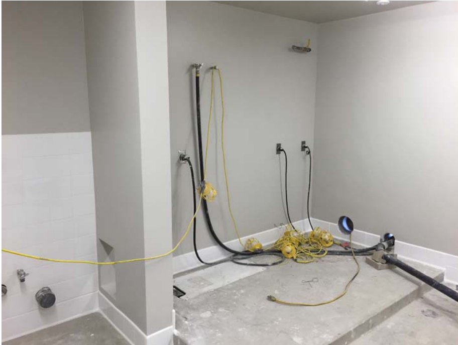
View of Laundry Area
