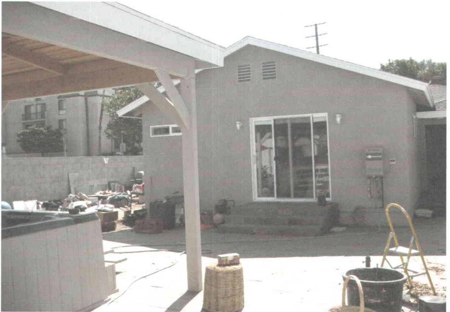
North view photo (rear view of new addition) photo taken on 04-21-11
