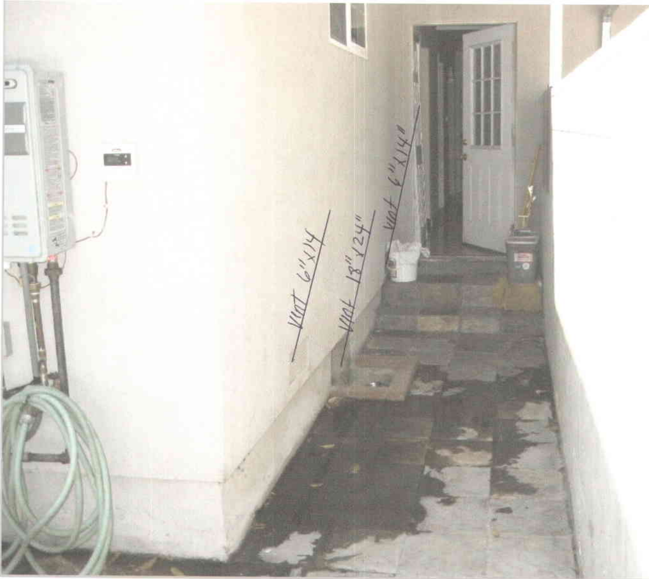
West side view photo taken date 04-21-11
