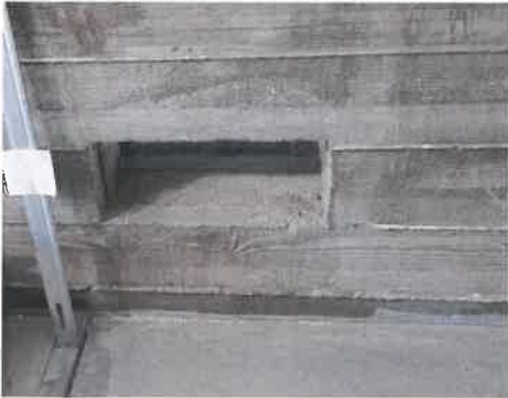
Garage- North wall ✓
