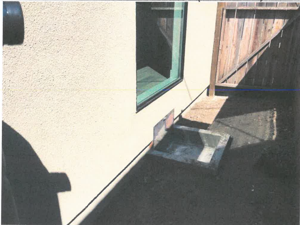
Photo Two Caption VENT / ACCESS AT REAR (ADDITION) EAST
