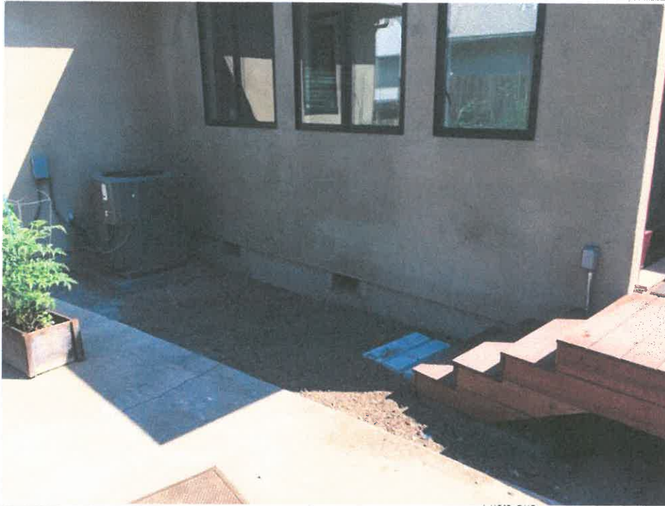
Photo One Caption VENTING AT REAR (ADDITION) WEST
