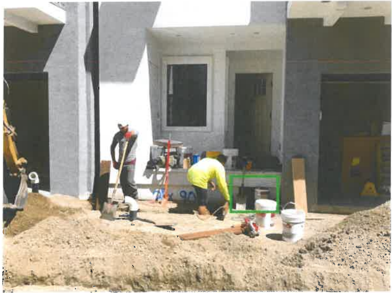
Photo 4: 04/17/18 Front of Home – Vent Under the Stairs. Before finished construction of Stairs
