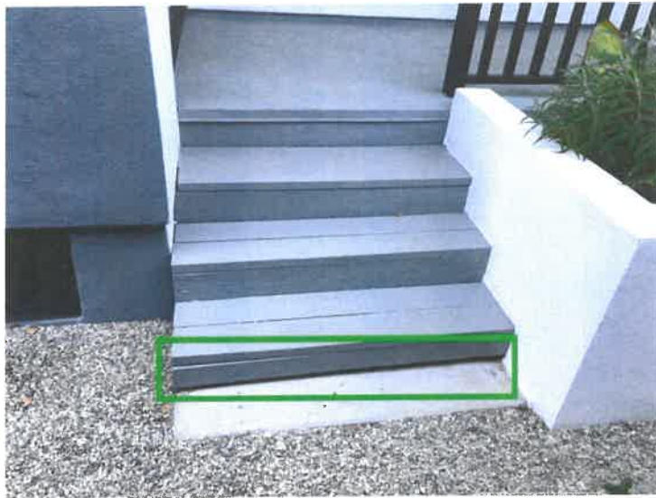
Photo 1: 07/13/18 Back-First Riser Open for Ventilation. Vent (12" x 18") behind the Stairs.
