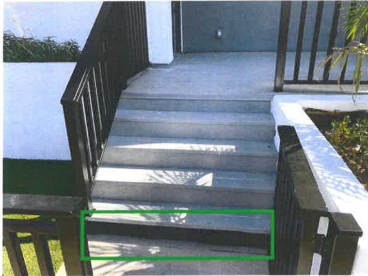
Photo 1: 07/13/18 Front-First Riser Open for Ventilation. Vent (18" x 24") behind the Stairs.
