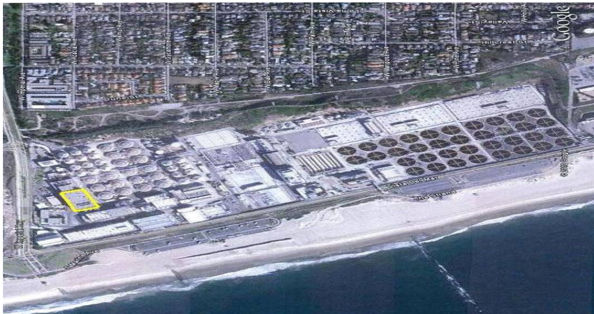
Figure 2. Current HTP Facility (potential project area shown in yellow).
